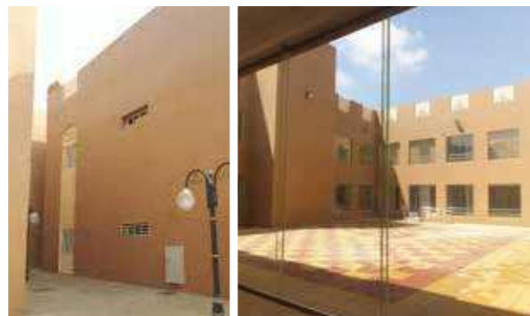
Construction of social care home complex for the elderly in Jazan region, Ministry of Human Resources and Social Development
