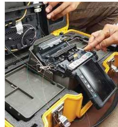
Fiber optics cable splicing for the Ministry of Interior between Riyadh - Makkah - Taif, Ministry of Interior
