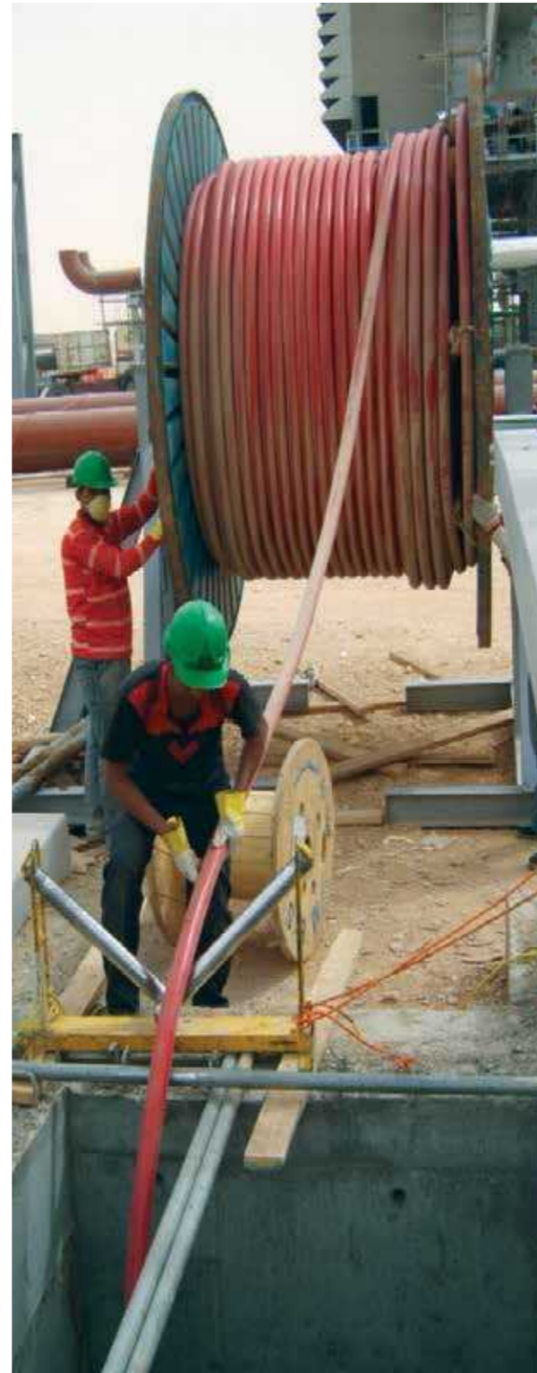
Extension of the electrical network, the Navy Jazan region
