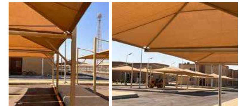
Construction of Breman facilities in Jeddah Air Defense Forces
